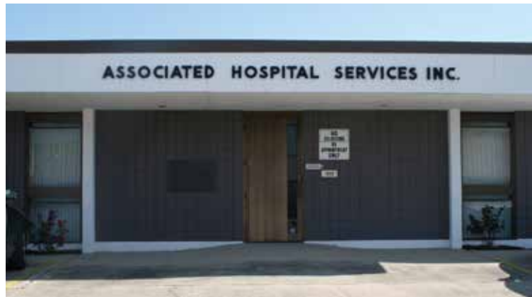
At left, nearly six years after Hurricane Katrina, scenes like this one in a middle-class neighborhood near the Associated plant unfortunately are all too familiar. Abandoned, storm-damaged homes stand alongside others that have been rebuilt. Above is the entrance to Associated Hospital Services.
